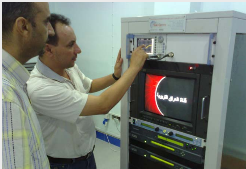
Setting the Transmission Unit
