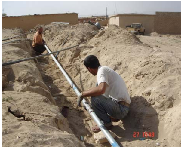
Men from tag-Harb Village installing water lines.
