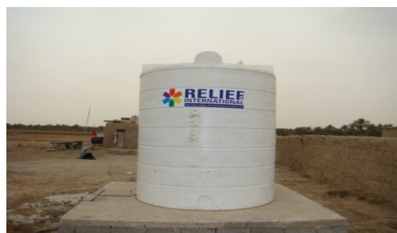
After - new water tanks throughout the village. Photos: RI
