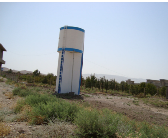
Water Storage Tank / Zavi Rash Village /KURDS
