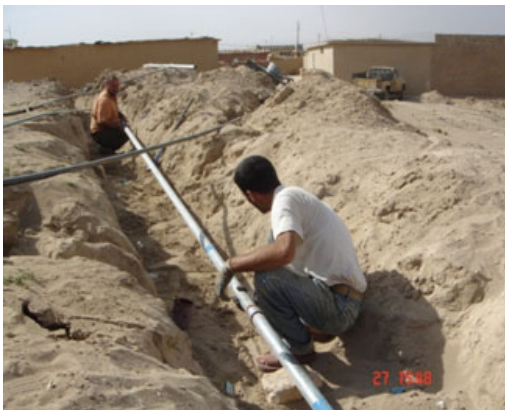
Men from Taq-Harb Village installing water lines.
