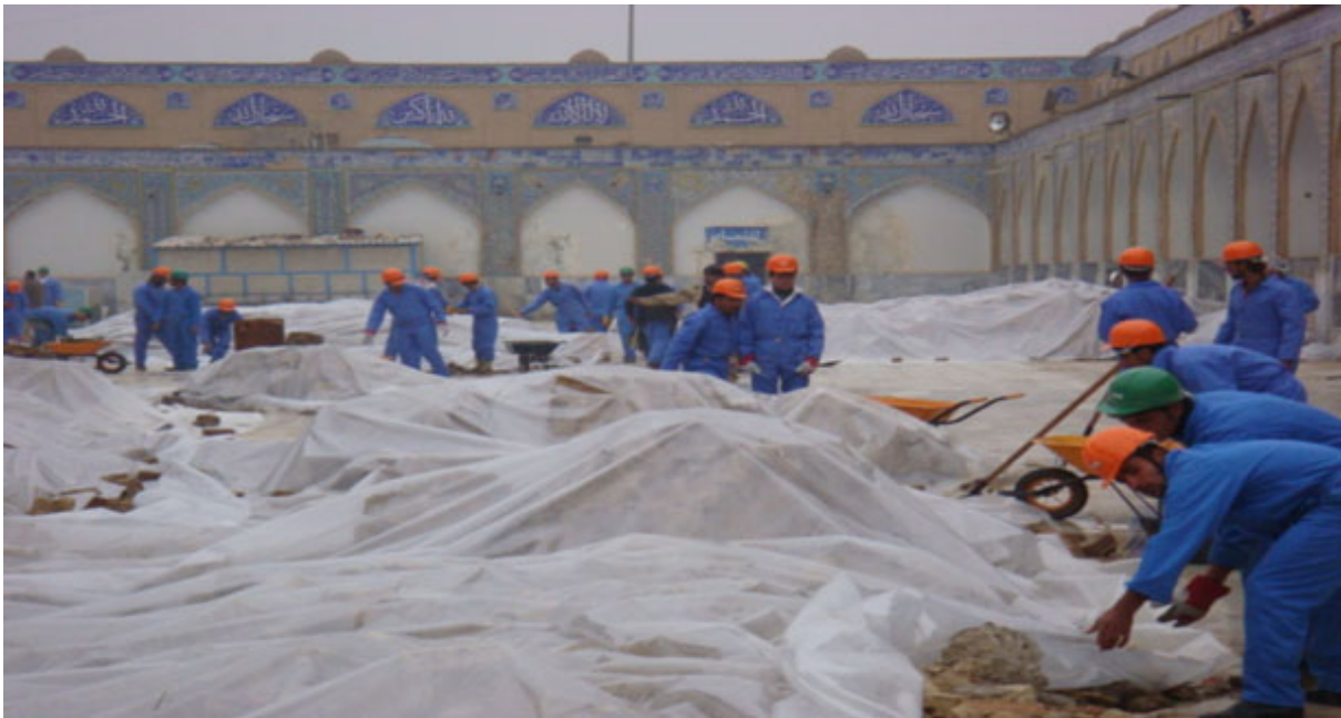
Protection of the ornamental elements scattered on the site
