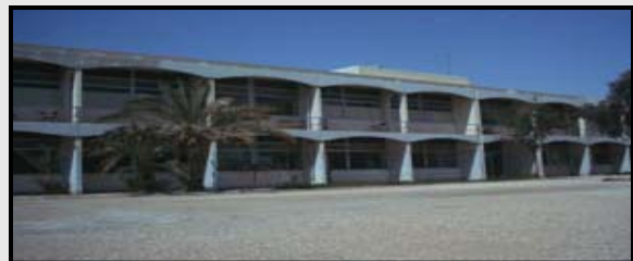
Nassiryah Facility Center/Training Workshop
