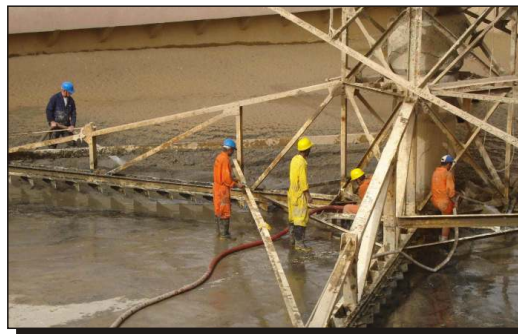
Cleaning and sludge removal from the Karama Clarifier
