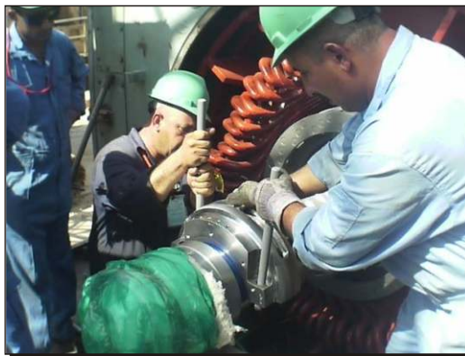
Taji: Installation of procured equipment
