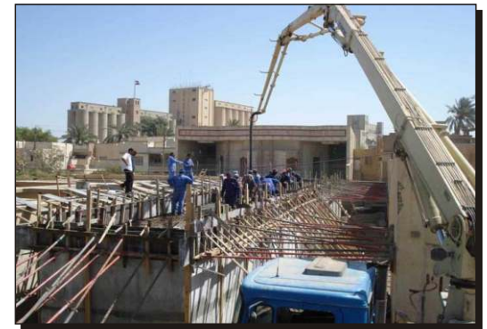
Construction of the roof on the new water tank in Karama
