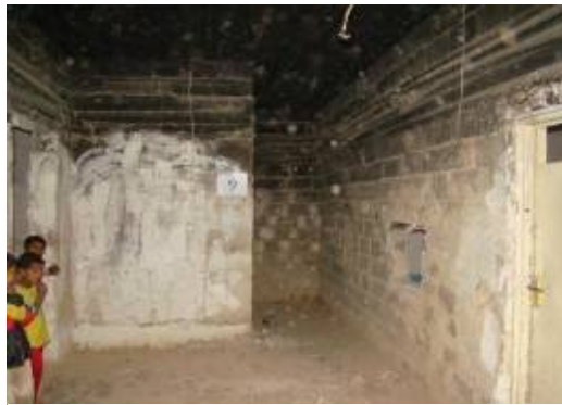
Faluja and Ramadi-Torched house interior before rehabilitation
