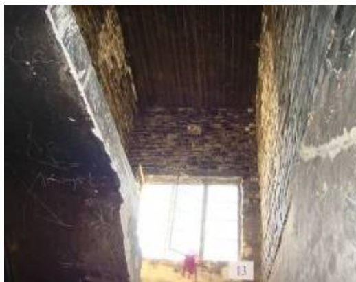
Faluja-House interior before rehabilitation
