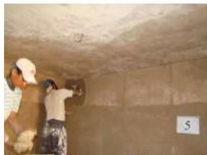
Shelter rehabilitation for returnees Falluja, Anbar – April 2009
