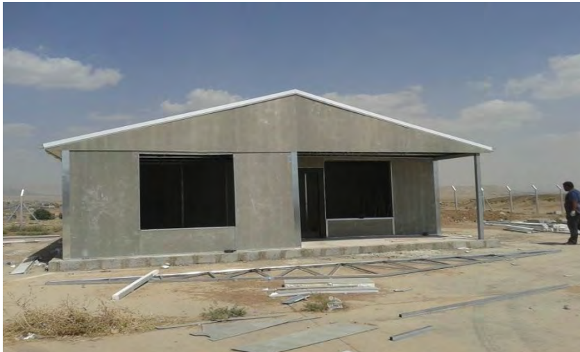
The construction of wedding rooms in Domiz-1 (UNHCR/ B. Amin)
