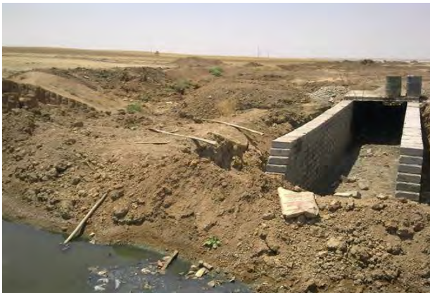
The construction of box culverts for the main drainage channel in Domiz-1 (UNHCR/C. Hungerbuehler)
