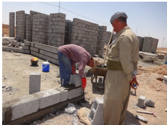
Construction of wall on the cement base © UNHCR/ S. Perera
