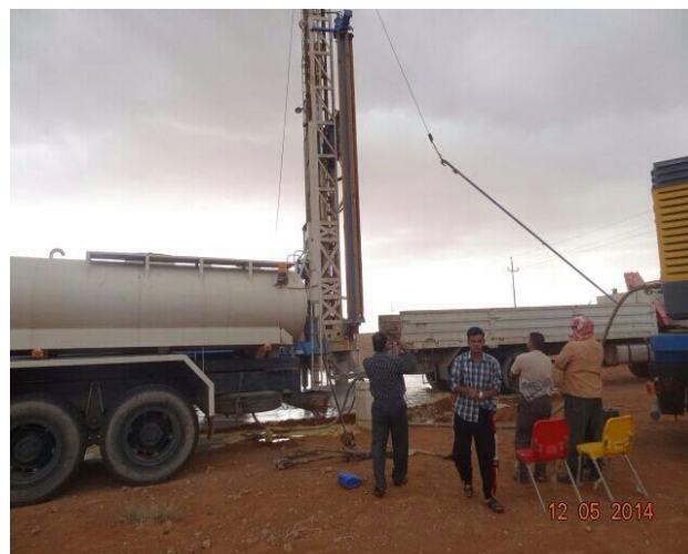
Digging of borehole in AL-Rutba-Anbar
